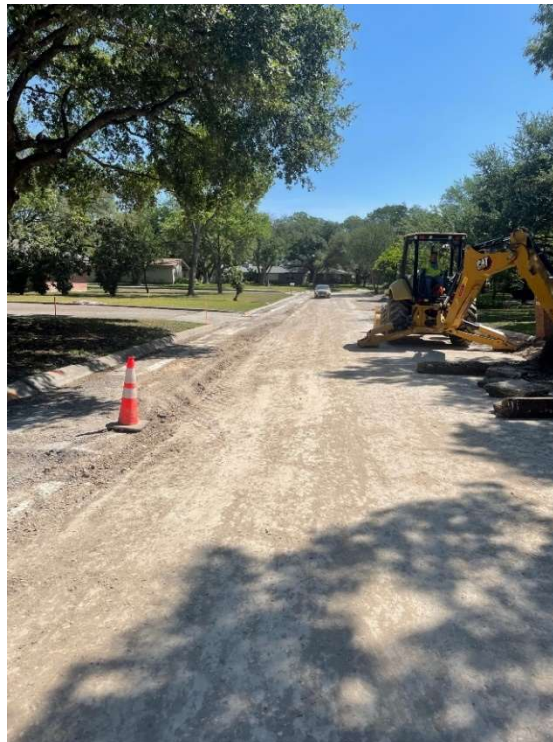
Figure 2: Briarcliff Dr. Full Depth Reconstruction
