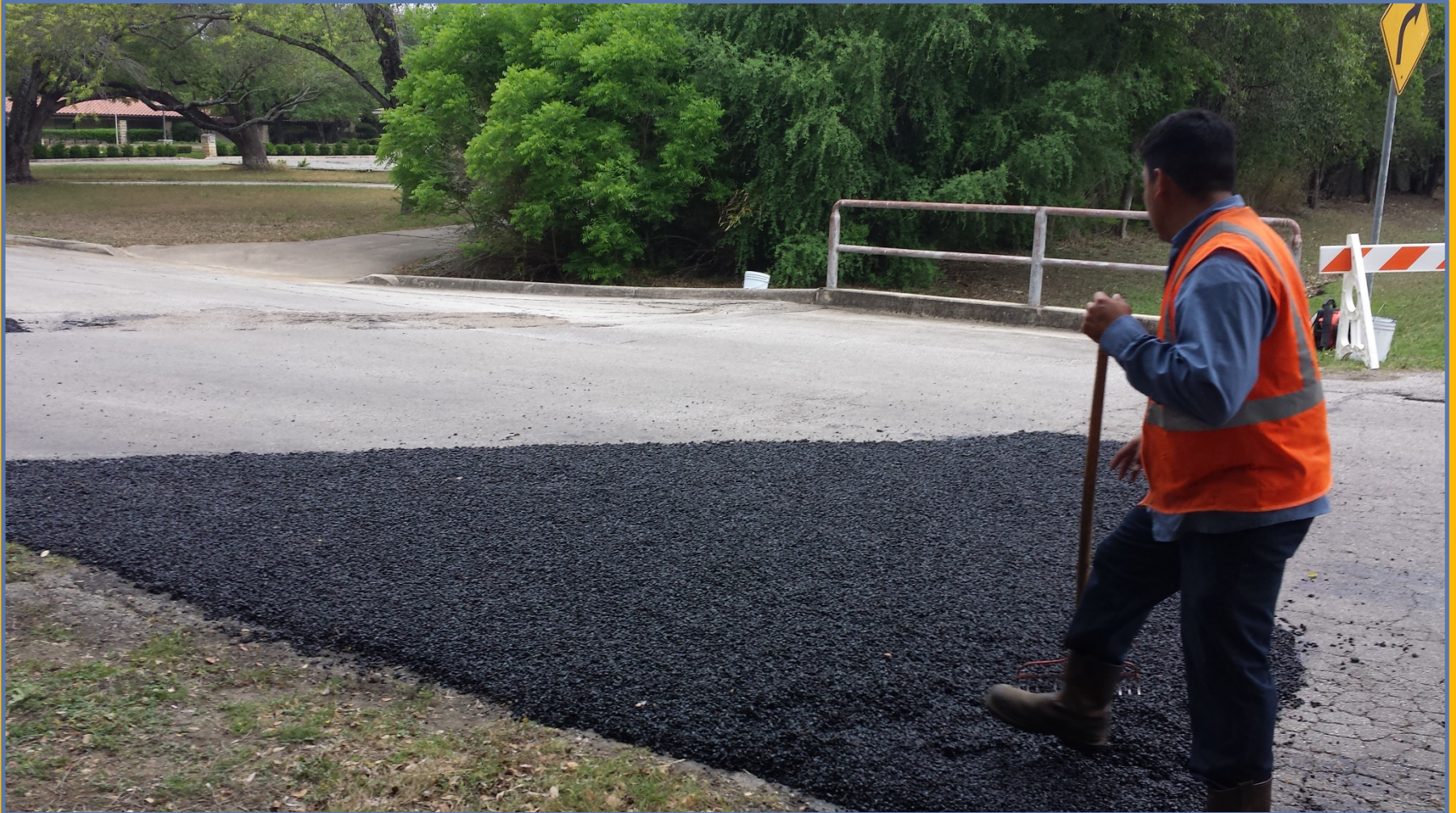
Application of UPM Cold Patch
