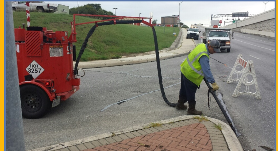
Crack Sealing
