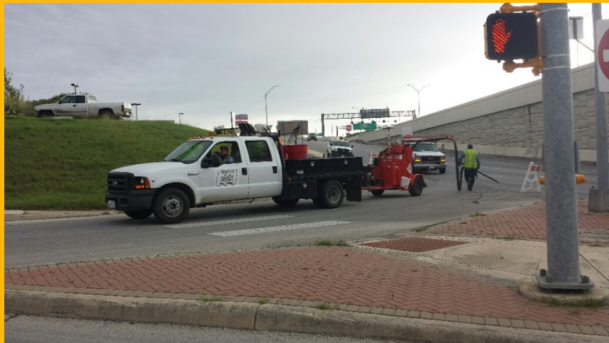
Crack Sealing
