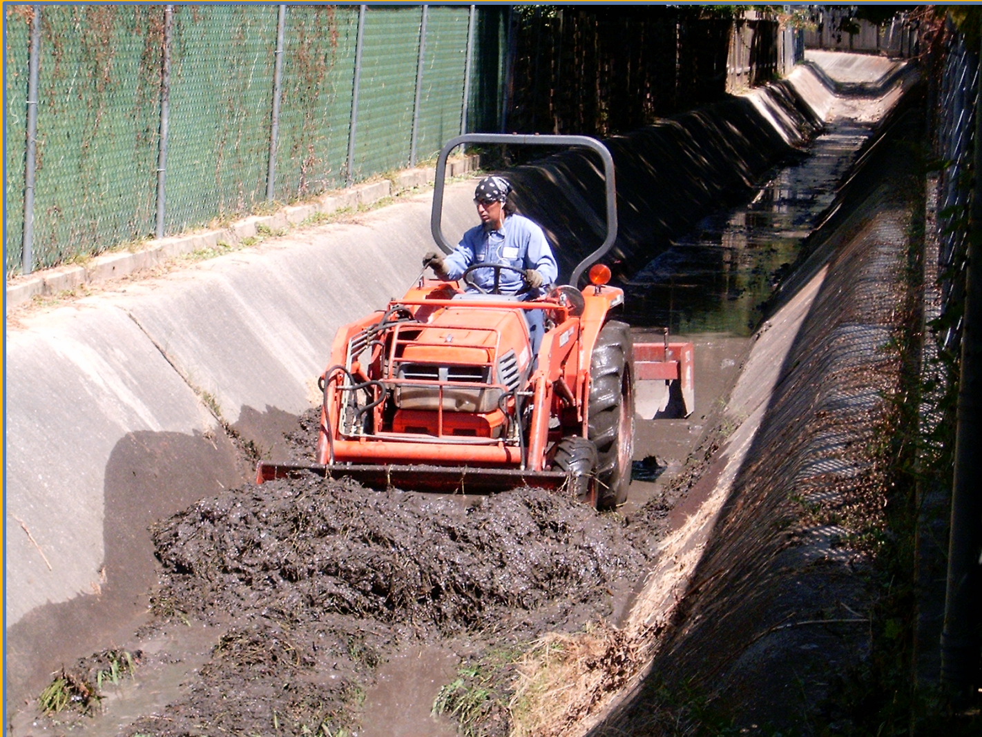
Cleaning out the drainage channel at Bluet
