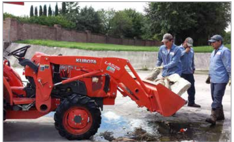
Public works employees work to remove broken concrete in the culvert behind the former Wedgewood apartments.
